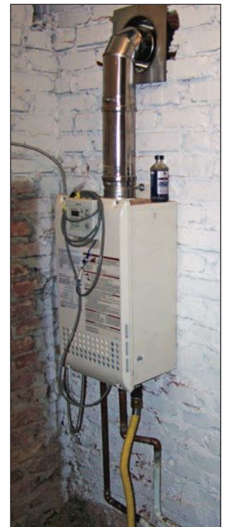
Figure 4: Tankless water heater (Atlanta, GA)
