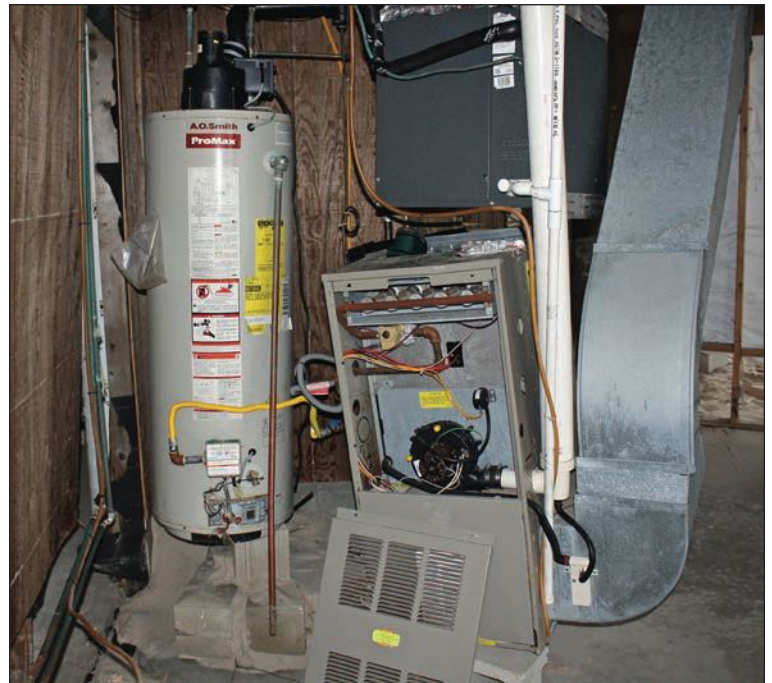
Figure 1: A water heater and furnace system damaged by Hurricane Sandy floodwaters (Beach Haven, NJ)
