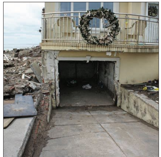
Figure 2: Coastal house with a below-grade garage and storage area, which typically contain utility systems. These areas are subject to flooding (Manhattan Beach, Brooklyn, NY).
