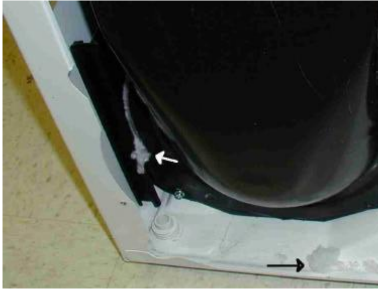
Figure 50. Lint Build-up at Blower Housing Seal and Dryer Floor
