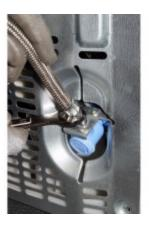
PHOTO: Disconnect the water supply line.
