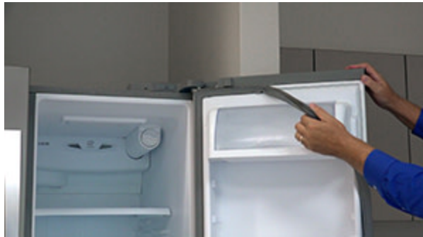
PHOTO: Remove the refrigerator door gasket.
