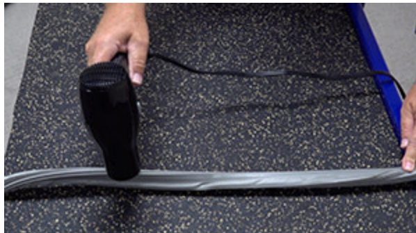
PHOTO: Remove creases in the new door gasket.
