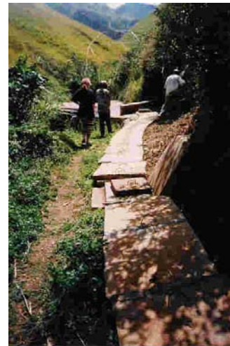
Covers to the roughing filter treating spring water, Eastern Zaire
