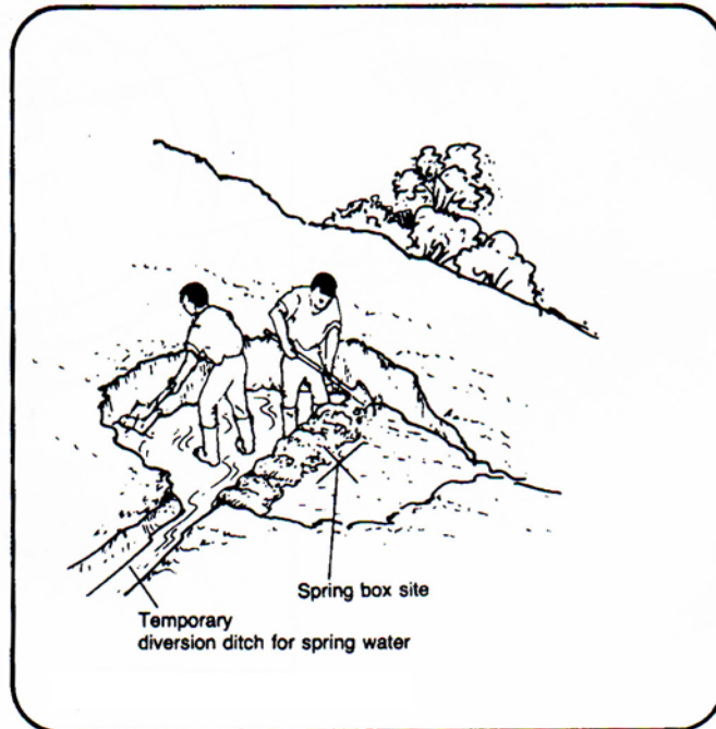
Figure 7: Excavating the spring site. Note temporary diversion ditch (Courtesy of USAID, 1982, available online at www.lifewater.org )
