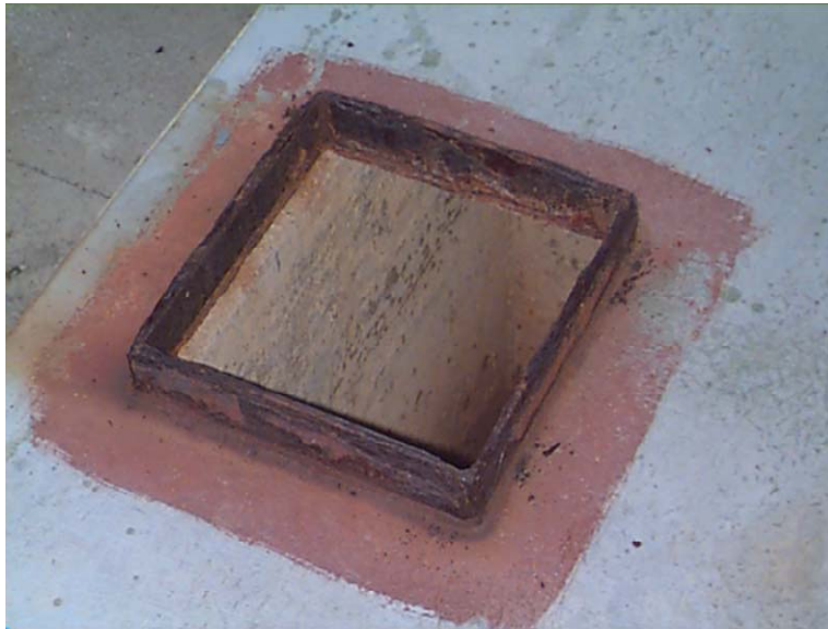
Exhibit 2.2 Raised Sill Appropriate for a Hatch
