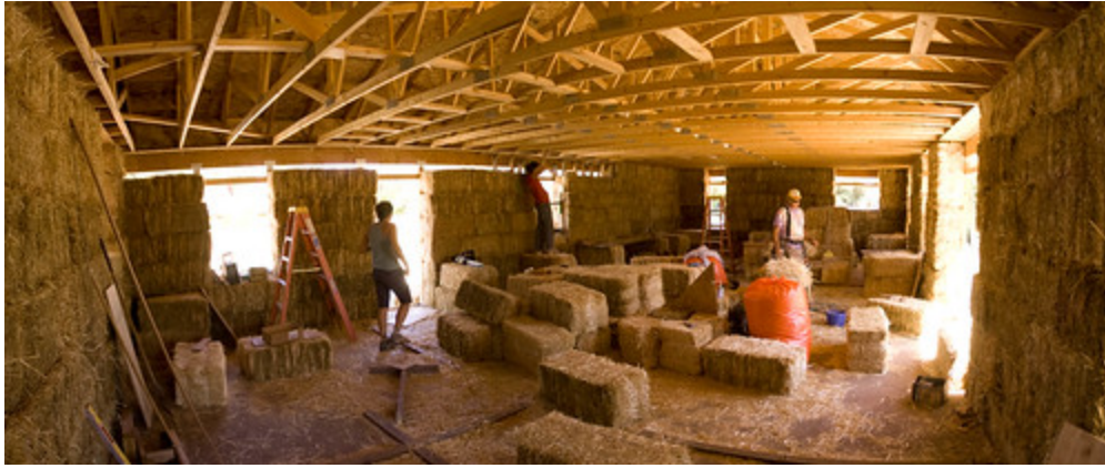
Construction of the straw bale home in Moab, Utah.
