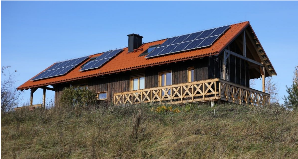
Figure 1. Single-family straw bale dwelling under study. Photo: Michał Pierzchalski.
