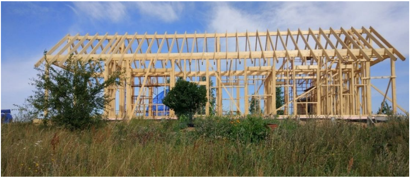
Figure 5. The timber structure of the building. Photo: Michał Pierzchalski.
