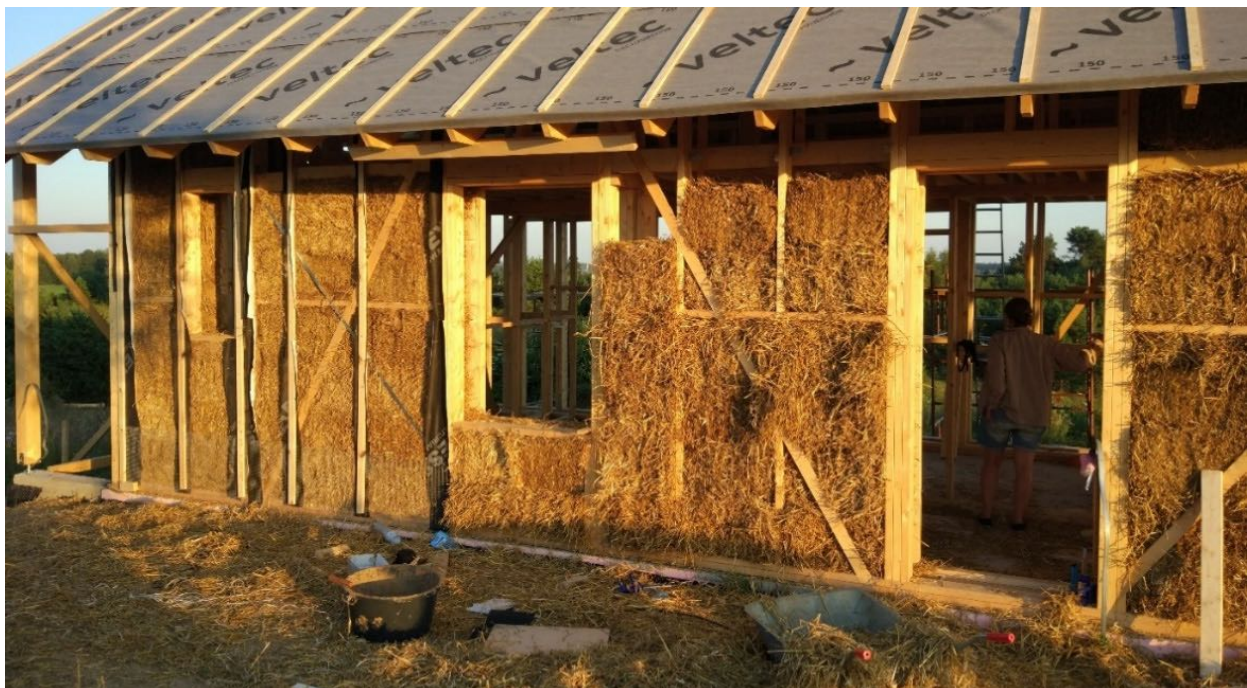
Figure 6. Outer wall filled with bales of compressed straw. Photo: Michał Pierzchalski.
