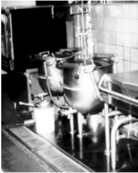
Fig. 5. Area under food preparation equipment is raised above a smooth stainless steel floor, allowing for easy cleaning of food spills and open to prevent harborage.
