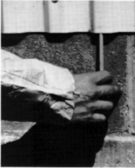
Fig. 12. Metal siding may provide entry points for mice and rats where panel ends are left open (left). Properly installed metal siding rests on the concrete floor or has metal flashing or angle iron to block entry (right).
