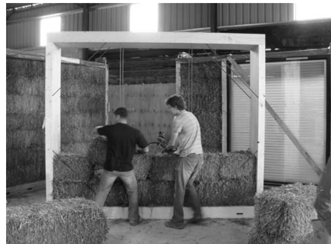
Figure 2. Panel construction process in ‘flying factory’
