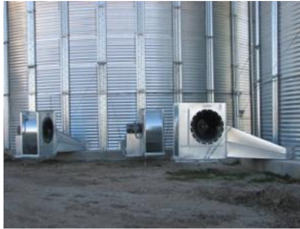
Bin aeration fan (photo: Feed&Grain.com)
