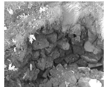
Figure 3. Collapsed Cesspool
