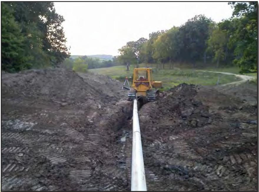
*In this picture, I am dragging the drain pipe in so I can bury it, Before I cover it up, I will put a seep plate around it.*
