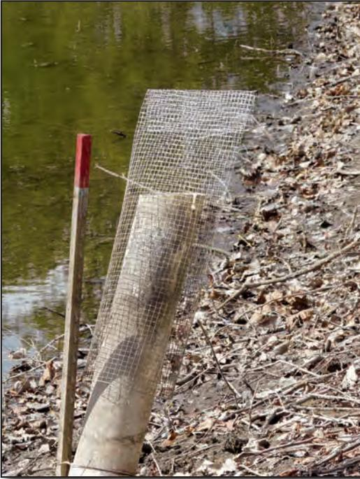
A vertical stand pipe or overflow like the above picture is the best and most effective. When the water level reaches the top of the pipe and runs over, the water will build up a suction or siphon effect and pull the water out. This is best on ponds that have a lot of watershed and can be quick to overflow.
