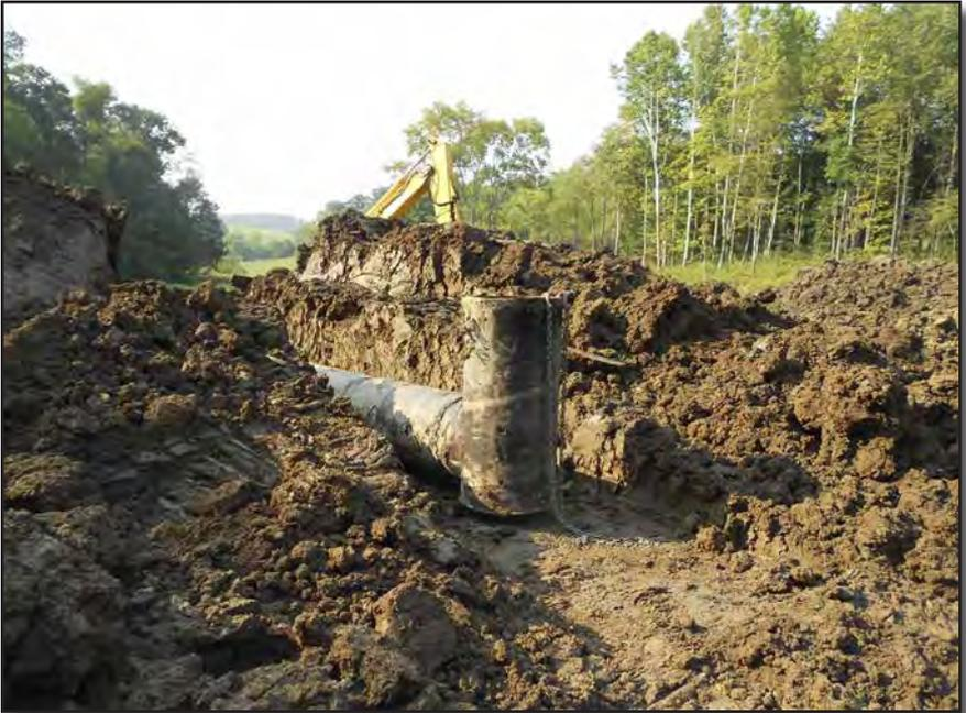
*This picture and the one below show a standpipe type of overflow.*
