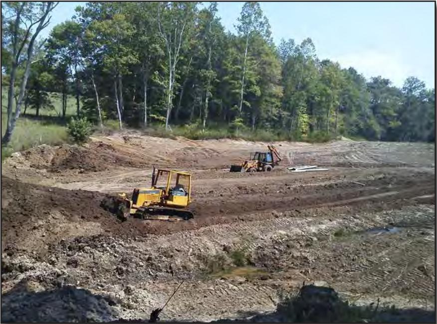
*In this picture, I am in the process of pushing the dam up. If you have some rain fall while you are building the pond, it will help to always keep some slope in the bottom so if it does rain, the water will drain away. If the water can't drain away, you will have a muddy mess.*
