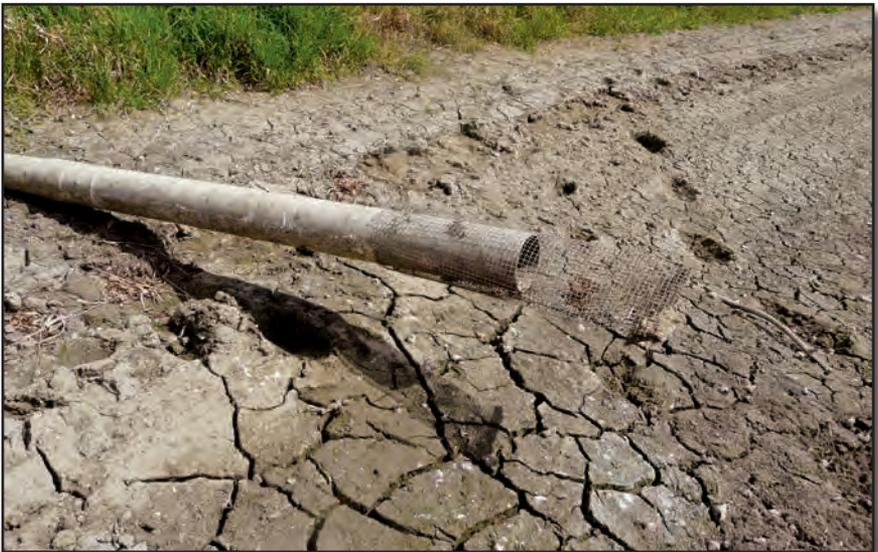
A horizontal pipe can't be used to its fullest potential until the pond level is too high. Unlike a vertical pipe, this type seldom will build a suction.
