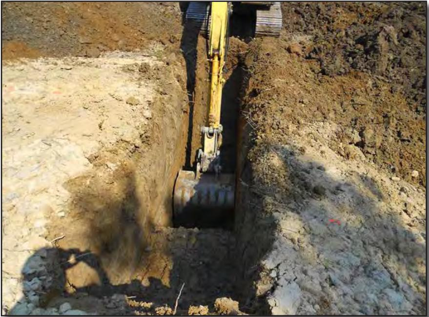
*Digging the core. One of the first stages of pond construction.*
