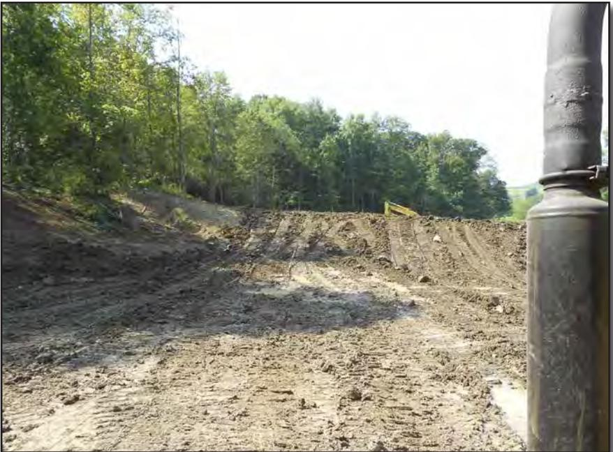
*Note that the bottom of the pond is smooth and uniform to provide drainage during construction.*
