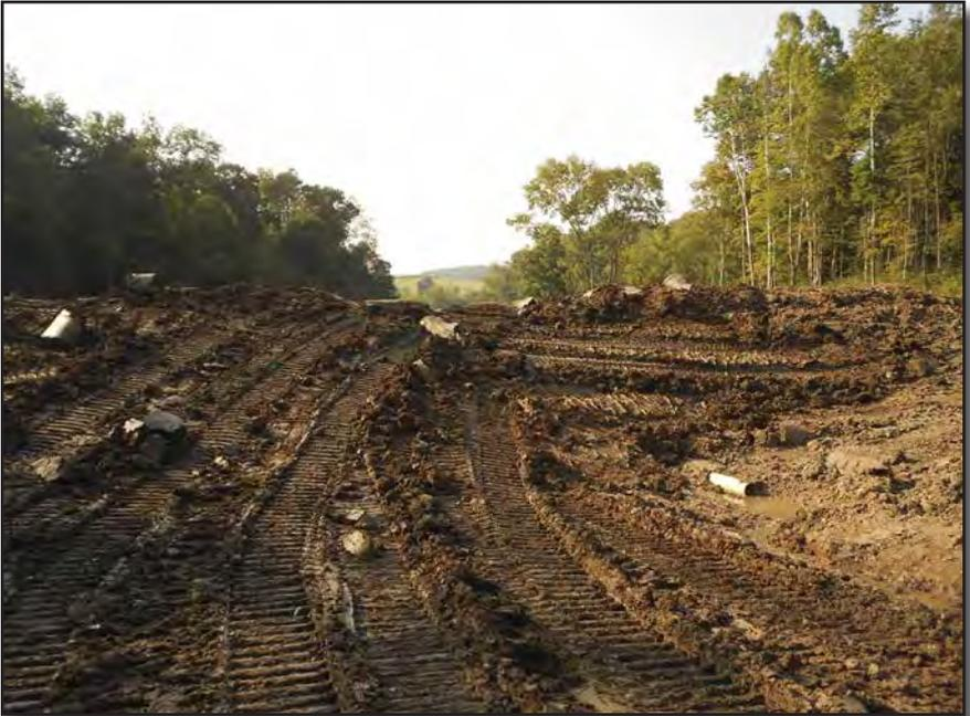
*The picture on this page and the ones on the opposite page show the final stages of dirt back on the dam after the pipes have been installed.*
