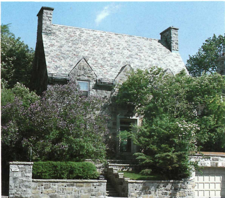
73* 1291 Redpath Crescent, Montreal, 1928. Architect of both houses: H.L. Fetherstonhaugh
