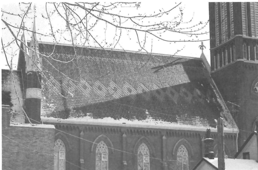
22 Welland Avenue United Church, St. Catherines, Ontario, 1877
