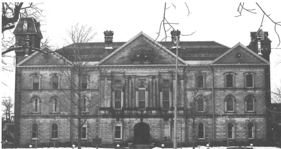
49 Brant County Court House, Brantford, Ontario (1852-53); polychrome slate roof added 1886
