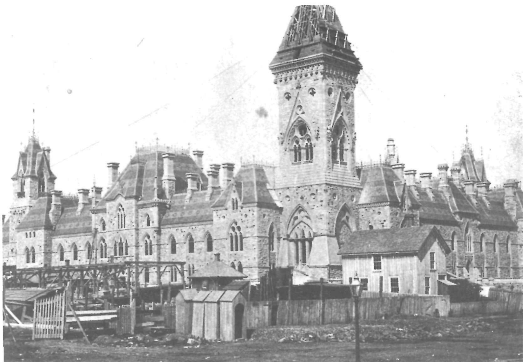
81 East Block construction 1862-64. Note board sheathing on tower. ( National Archives, C-37299 )
