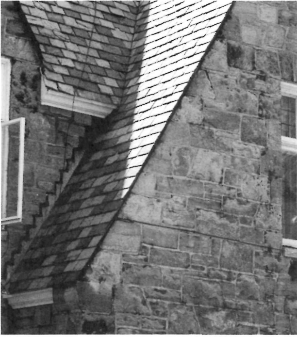
84 Base flashing running under slate
