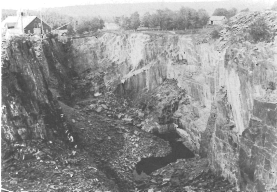
93 Melbourne slate quarry, Eastern Townships, Quebec ( National Archives, PA-40112 )
