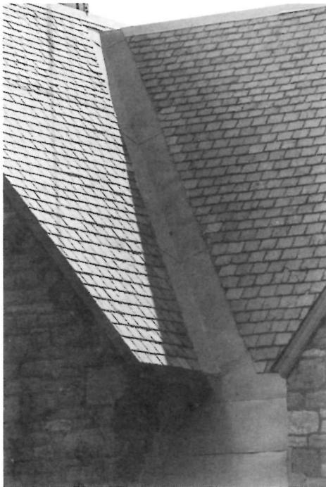
86 Open valley with wide flashings, typical of most Canadian slate roofs
