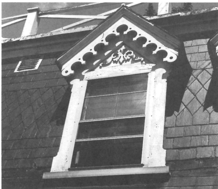
40 Mansard slate designs: 168 Jackson Street, Hamilton, (top) and 165 Moore St., Sherbrooke, Quebec
