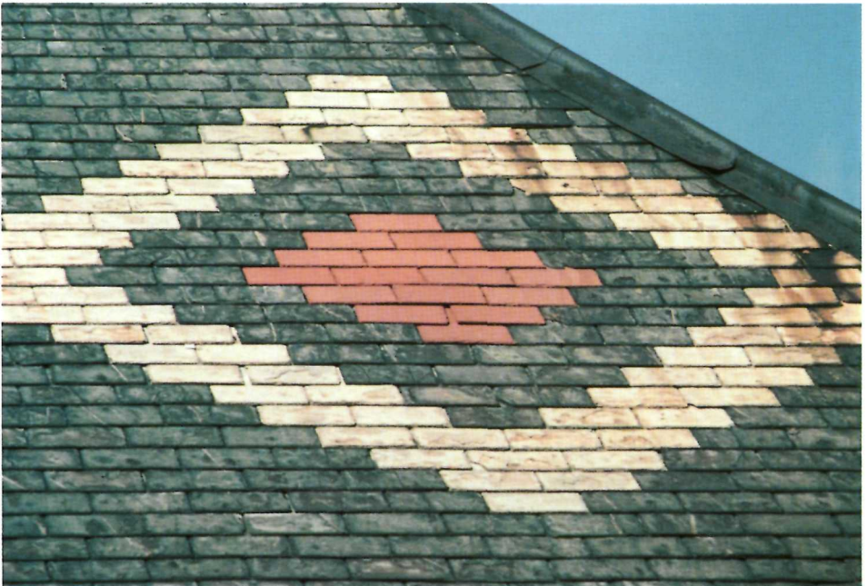
88* Galvanized iron flashing, Wellington Street United Church, London, Ontario, 1878
