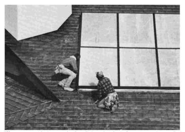
"New copper shingles can be installed easier than almost any other roofing method. Just snap two copper shingles together, and then put in two copper nails. No highly skilled craftsmen are needed," says the principal architect of this Denver home and member of the legendary Wright Foundation.
