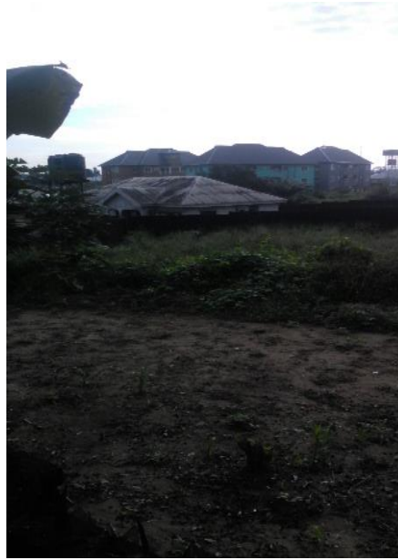
Fig. 4. The Roof Top of the Building in the Front is covered with Dark-Black Deposit, the Storey Buildings Behind are Roofed with Dark-colour Roofing Sheets to Conceal the Effect of the Dark-Black Deposit.
