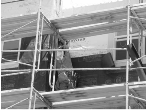
Illustration 1: Installing WRB at Corners
