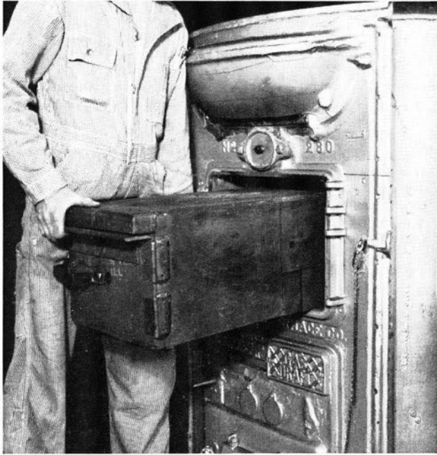
FIG. 23. DOWN-DRAFT BURNER BEING INSTALLED IN FURNACE
