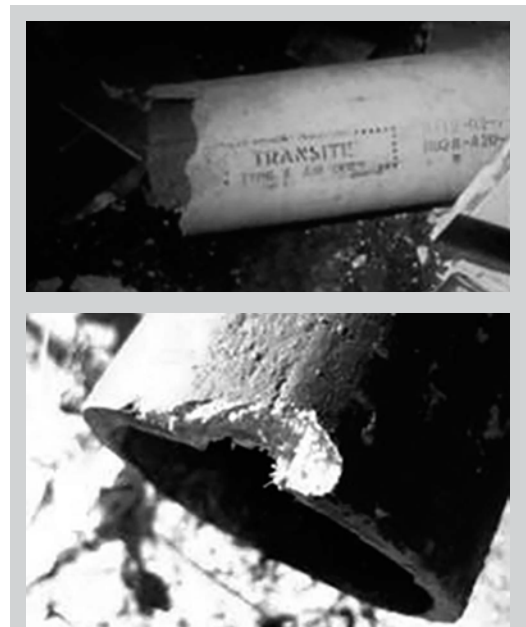
Figure 5: AC pipes usually contain anywhere from 10 to 75 percent asbestos.
