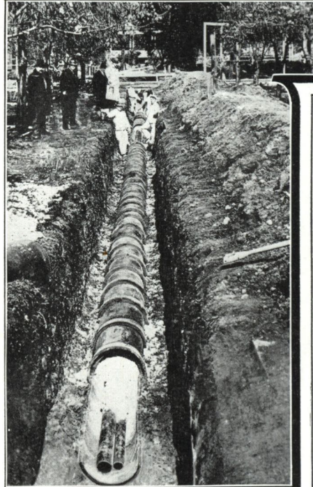
Above - Pipes being insulated before top of system is applied at Battle Creek Sanitarium Battle Creek, Mich.
