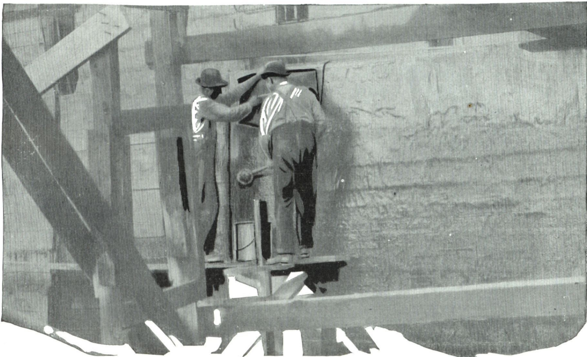
Applying Johns-Manville Waterproofing on side walls. See detail drawings on page 200.
