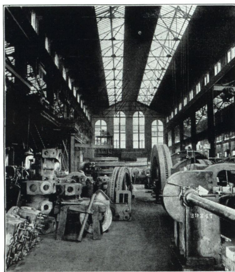
Demands of extremely heavy duty being satisfactorily met by Johns-Manville Industrial Flooring in the shop of the De La Vergne Machine Co., New York.
