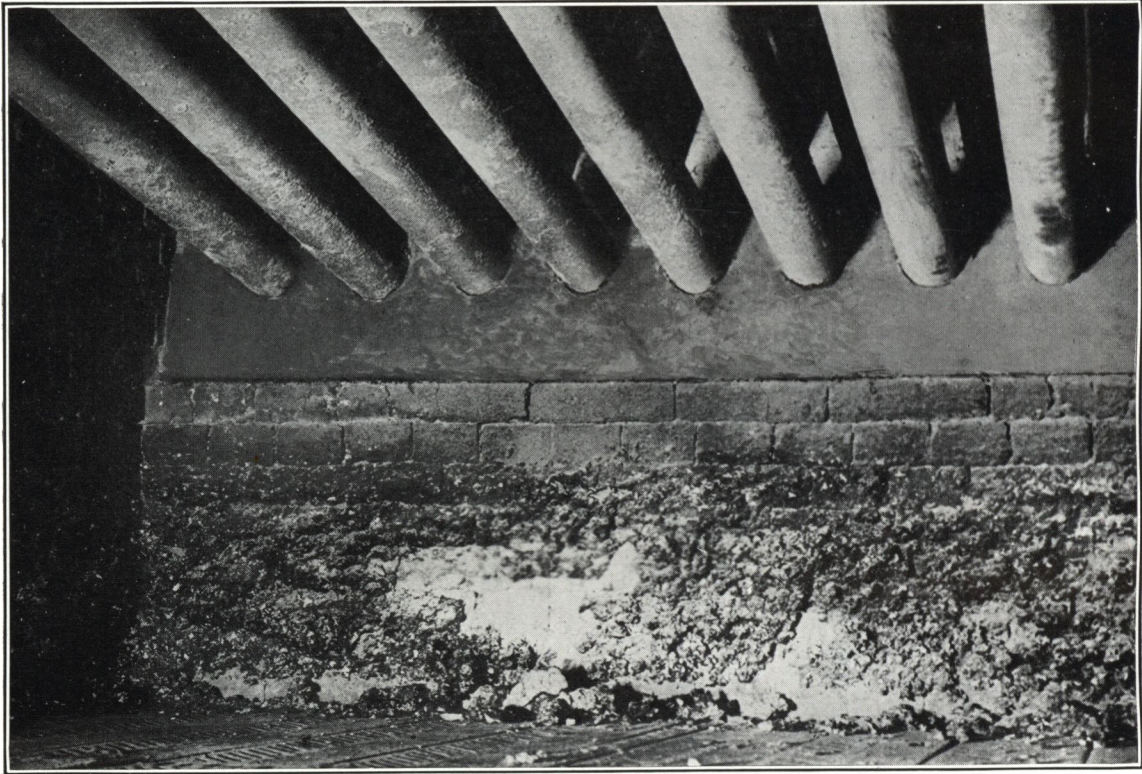
This is an excellent illustration of the Johns-Manville Monolithic Baffle Wall, showing as it does, a solid wall built up around the tubes, with none of the joints and cracks necessarily found in tile baffle walls. It can readily be seen from this picture that leakage of heat-laden gases through such a wall is absolutely impossible, as it is built of a material that will resist and withstand highest temperatures encountered without melting or cracking
