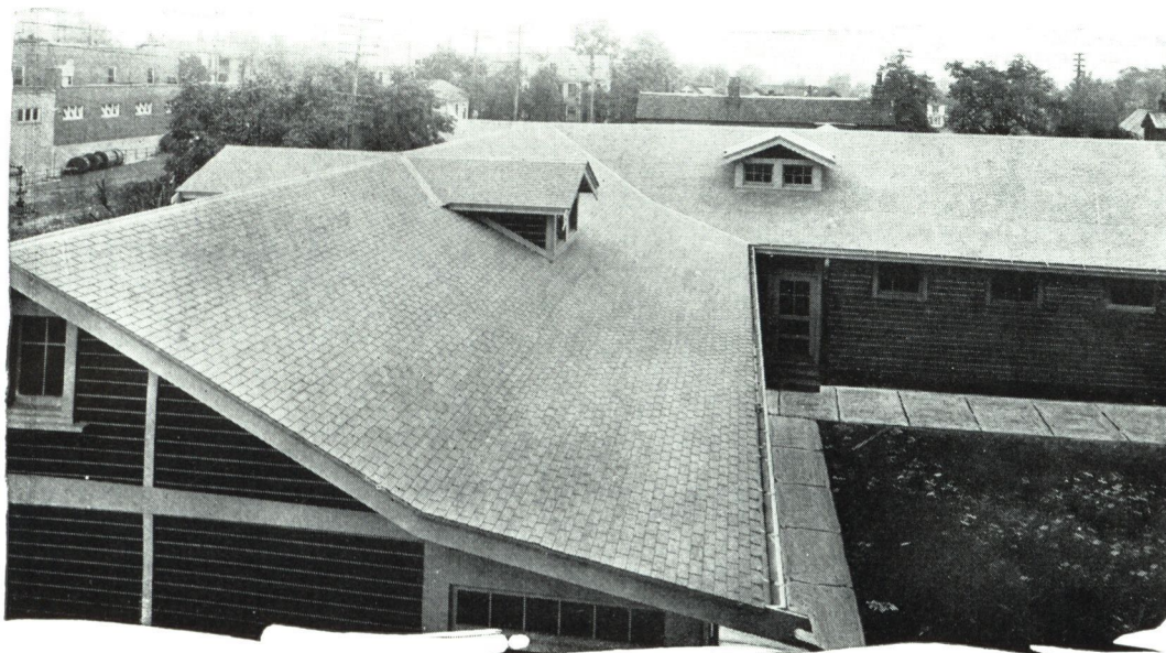
Flexstone Asbestos Shingles afford better service and greater fire protection because of their all-mineral, asbestos rock fibre felt base.
