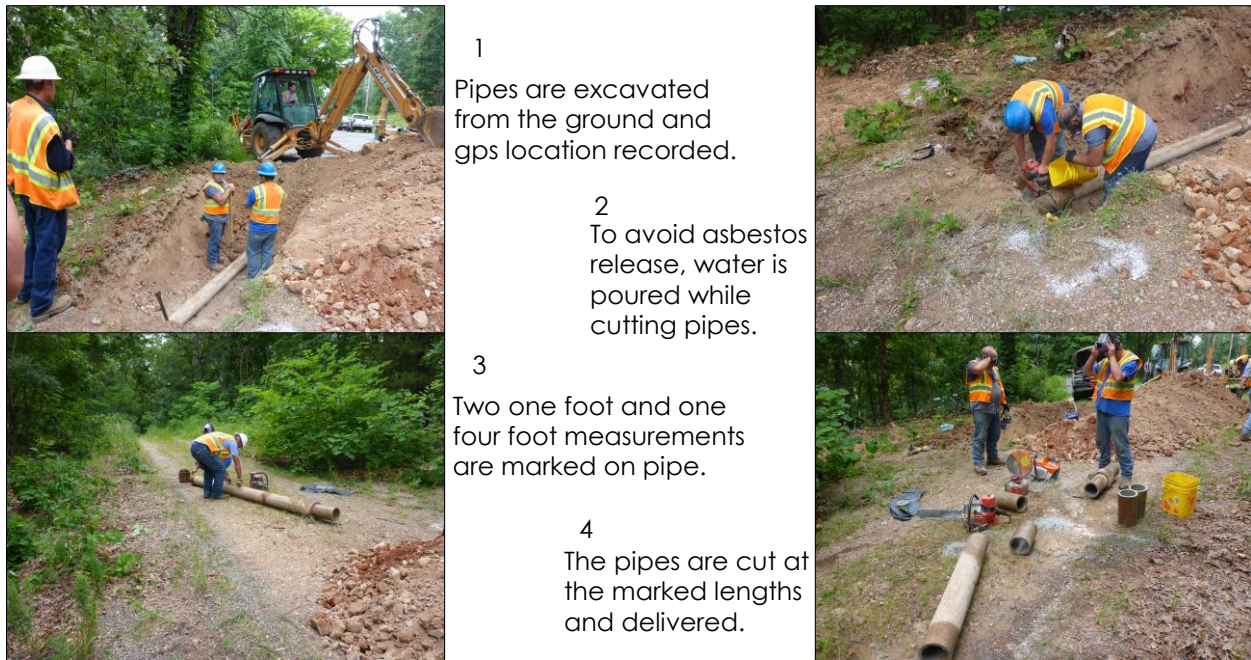
Figure 3-3. AC pipe sampling procedure
