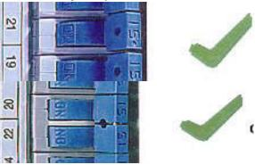
Check for a hole on the blue handle, as illustrated with check marks. Breakers with black handles are not an issue
