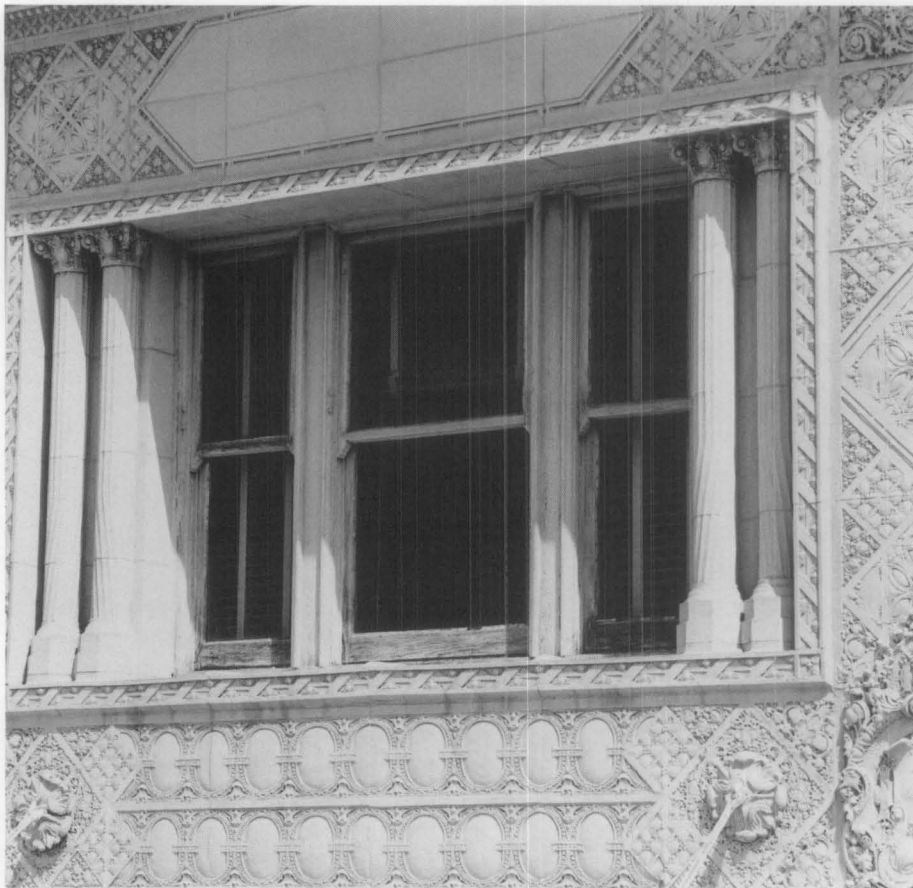
Figure 1. Deeply recessed windows with ornamental terra-cotta surrounds were character-defining features of the building which the owner wanted to retain. Photo: Jack Graves, AIA
