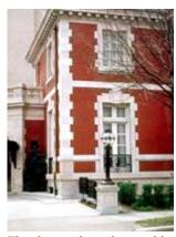
The decorative trim on this brick builing is architectural terra-cotta intended to simulate the limestone foundation. Photo: NPS files.
