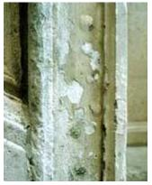
This clear coating has failed stone as it peels. Photo: NPS
