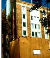
The lower floors of this historic brick and architectural terra-cotta building have been covered during chemical cleaning to protect pedestrians and vehicular traffic from potentially harmful overspray. Photo:
