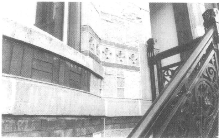
Figure 11. Close-up views of the newly installed pre-cast concrete units and the reinstated original brick. Photo: James Smith
