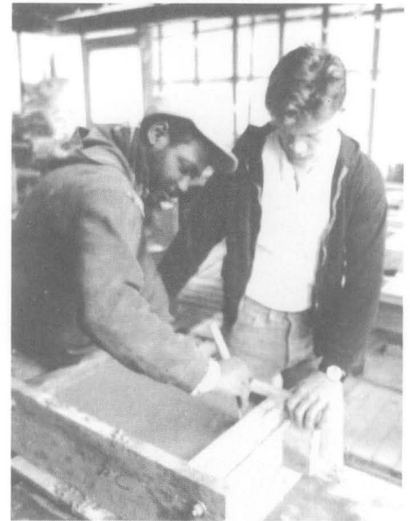
Figure 7. The workmen shown here are cutting the air bubbles from the sides of the mold using a cake spatula during the first 10 seconds of the vibration process. Photo: James Smith
