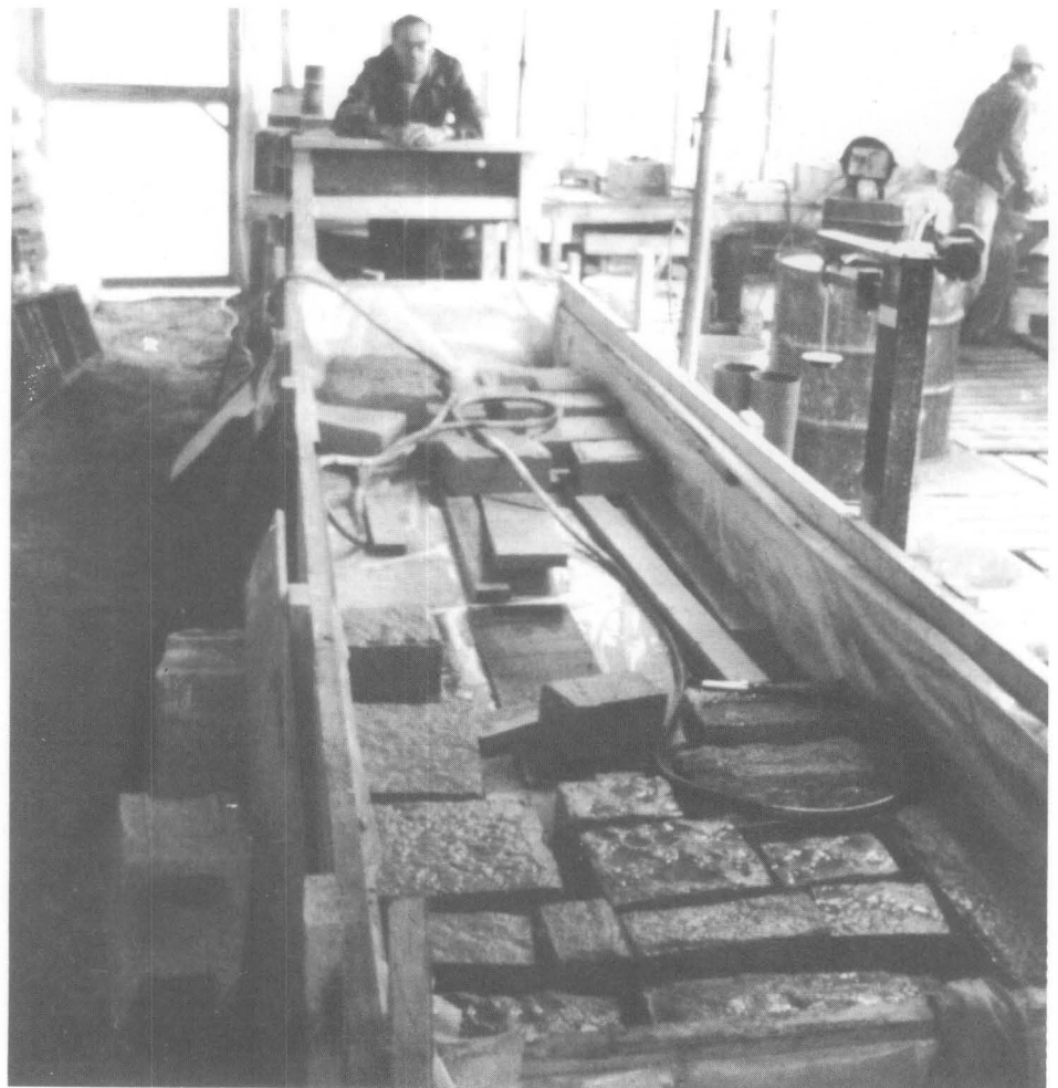
Figure 8. After soaking for 6 hours to remove soluble salts in a polyethylene-lined wood water tank, the pre-cast units were allowed to dry for another 6 hours. This process was repeated 3 times for each pre-cast unit. Photo: James Smith
