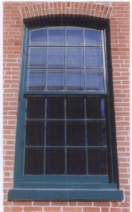
Figure 7. The new window's joinery, individual glass lights, reflective qualities, and painted wood finish all help to capture the appearance of the original units.
