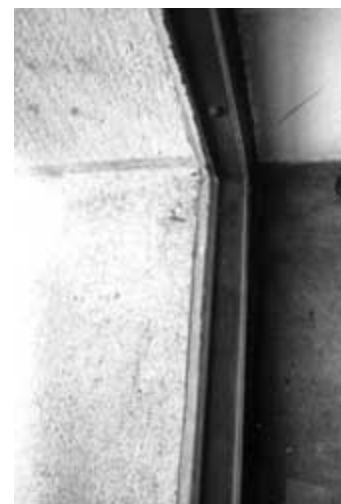
This is a successful replacement in kind of the deteriorated frame shown above. Photo: Henry Chambers, AIA.
