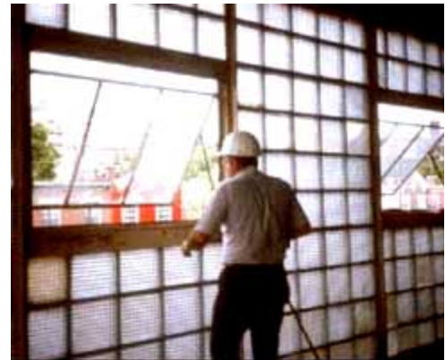
Maintaining historic steel windows for continued use is always recommended.
