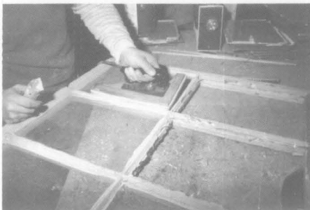
Figure 3. Electric deglazing irons were used to remove hardened putty so glass could be removed and the sash frames repaired. Photo: Christopher Closs
