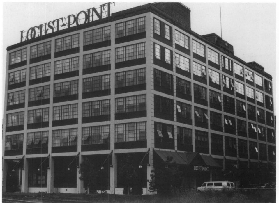
Figure 13. Lippincott Press Building (now Locust Point) after repair of the multi-light steel windows. Photo: Robert Powers.
