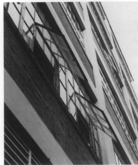
Figure 7. Retrofitting projecting ventilator with the TRUTH hinges. Photo: Robert Powers.
