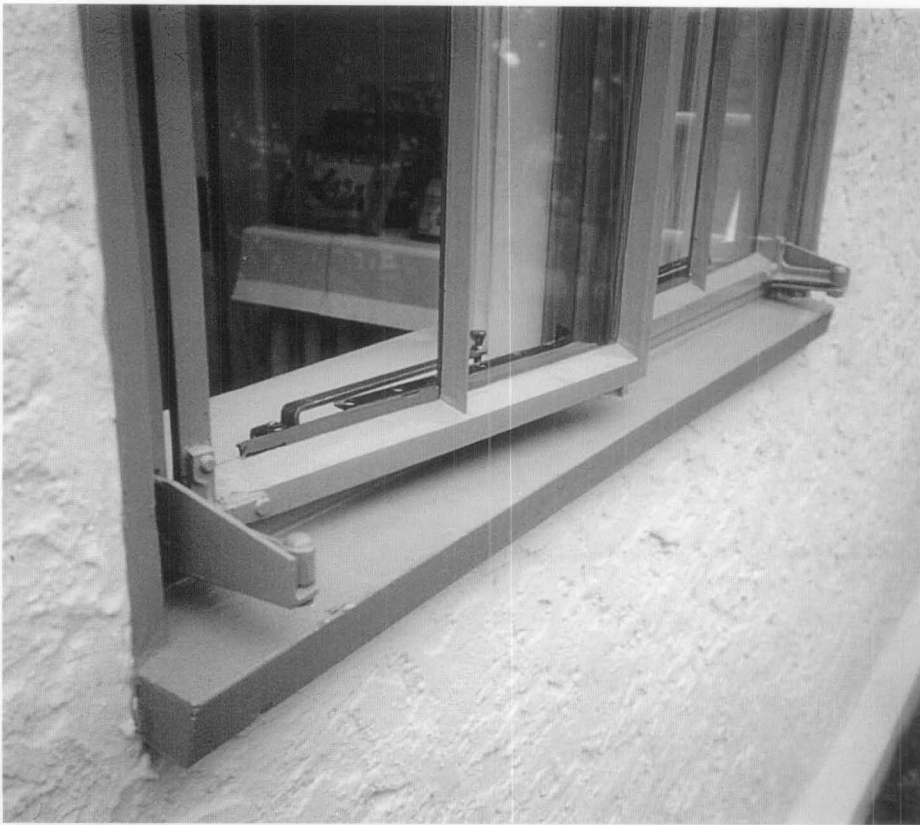
Figure 10. Detail of complete windows, repaired, serviced, reglazed and repainted.
