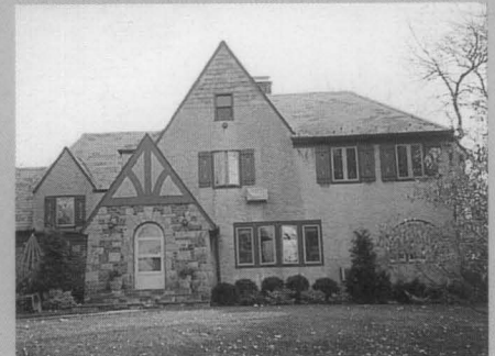
Inappropriate replacement windows dramatically affect the appearance of a historic home that once featured steel casement windows.
