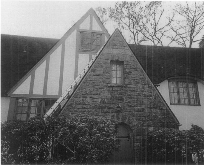
Figure 1. Steel casement windows were placed in various configurations throughout the house. Grouped windows open in opposite directions from each other, assuring that breezes can be captured, and a sash opened during rainy weather, regardless of the wind direction.
