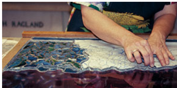
Figure 14. The external glass plate has been removed to clean the interlayer of this plated Tiffany Studios window.
