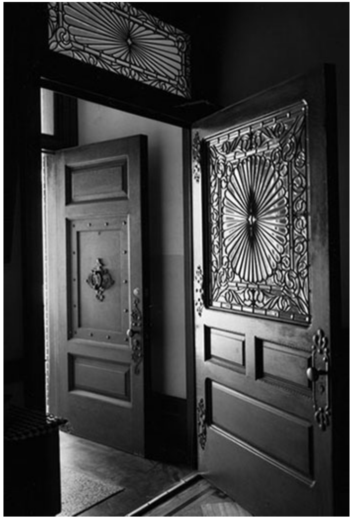
Figure 1. This door and transom suggest the richness of 19th century leaded glass. Photo: Jack E. Boucher, HABS.
