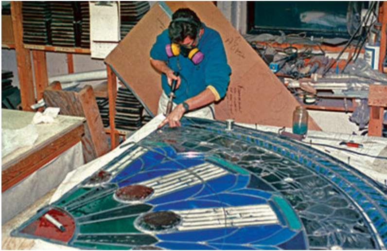
Figure 17. Total releading is very time consuming and costly and should only be undertaken when the original lead is exhausted beyond repair.
