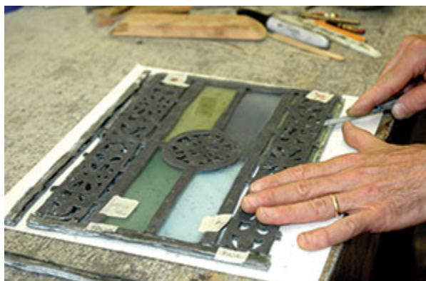
Figure 15. To permit repair of the cracked glass, the original lead overlay is first salvaged from this historic leaded panel of silhouette glass to retain as much of the original work as possible.
