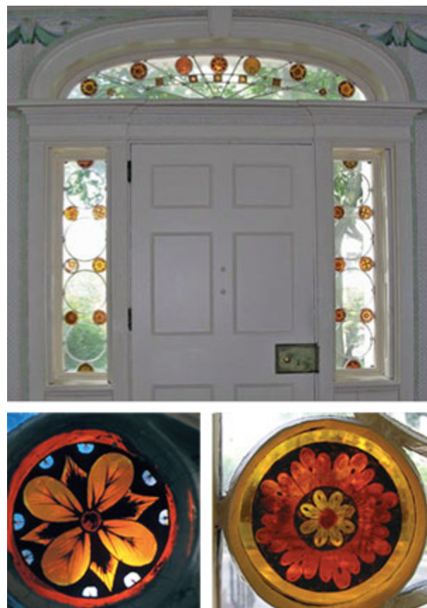
Figure 3. The entrance to the Morris-Jumel Mansion, New York City, is one of the earliest surviving installations of stained glass in the country. It features a fanlight and sidelights of large clear roundels and small bulls-eyes of red and orange glass tinted with silver stains from ca. 1810. Photo: Ken Moss.
