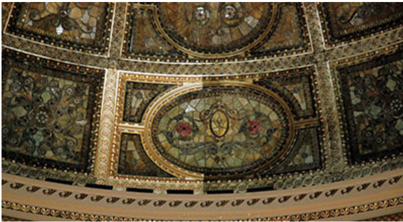
(a) Stained glass ceilings and domes are often principal interior features of churches, hotels, restaurants, railway stations, and civic buildings. This vaulted ceiling illuminates the Cypress Lawn Memorial Gardens mausoleum in Colma, California. The panel removed reveals the diffusing skylight above.
