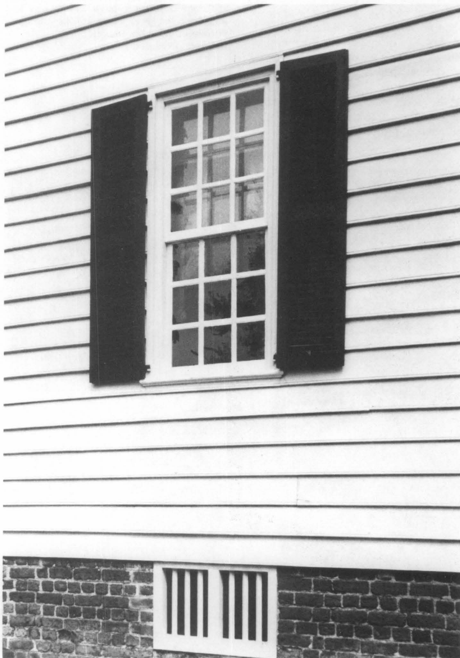
Figure 8. The unobtrusive interior storm window required no physical damage or exterior visual alteration to the original window. Photo: Tom H. Taylor.
