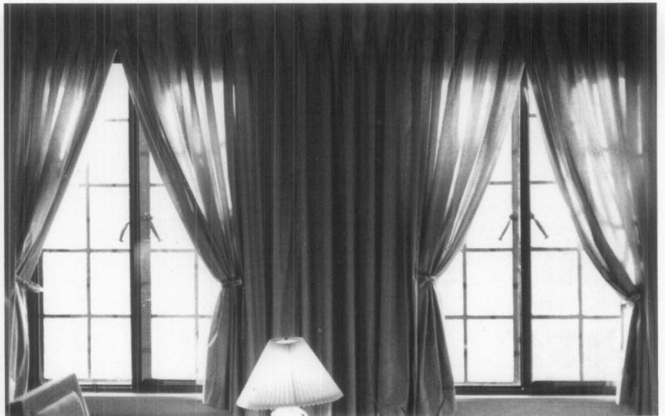
Figure 8. The storm units are neatly set within the opening and aesthetically are not disruptive. Photo: Charles Fisher.
