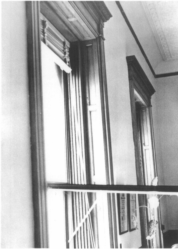
Figure 5. The interior storm window was designed to fit within the existing wooden jamb. The large size of the windows necessitated the use of operable storm panels, intersecting at the historic meeting rail. Here the lower storm panel is in an opened position for cleaning. Photo: Charles E. Fisher
