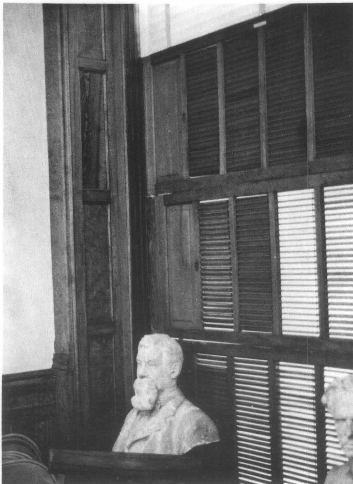
Figure 7. Continued use of the unique shutter system required that the frame of the interior storm window be narrow. The storm windows are set between the shutters and the historic sash. Photo: Charles E. Fisher
