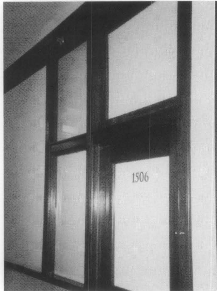
Figure 5. Completed Reliance Building corridor showing historic door panel, sidelight and transom. Photo: Chad Randl.
