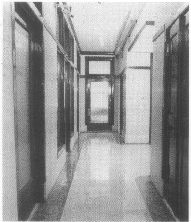
Figure 1. Historic corridor features such as doors, transoms and sidelights often do not meet current fire resistance regulations. Photo: Fisher Building, Frank Merrill Photography.
