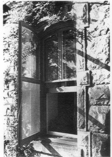
Figure 5. The new wooden storm sash was installed in the historic frame; the edge of the storm frame was rabbeted to accommodate the historic molding on the old wood frame. Photo: Richard Bierce, AIA
