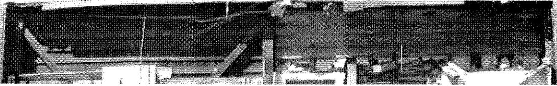
Figure 19: Beaded siding across top of recently-exposed rear elevation.
