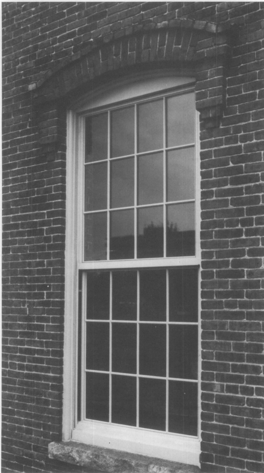
Figure 7. Replacement window after installation. Photo: Charles Parrott
