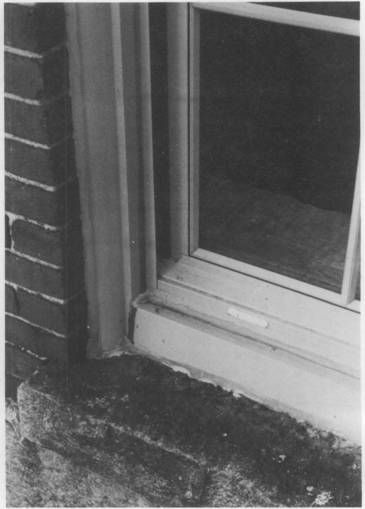
Figure 6. The manufacturer's stock window used for the project unfortunately created the appearance of a double sill, which the historic window never had. Photos: Charles Fisher
