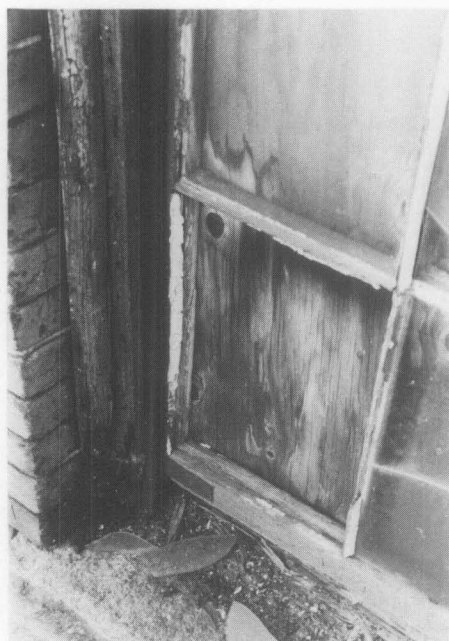
Figure 2. The condition of the windows varied considerably. Shown here is a typical case where the frame, sill and sash were beyond repair. Photo: Charles Fisher
