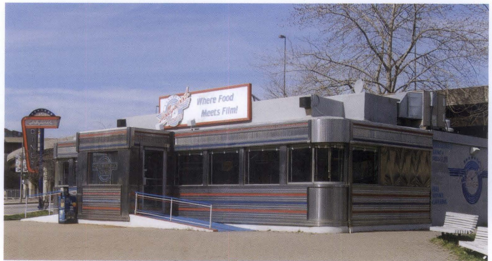
Figure 10. The shine and luster of an aluminum window with an original mill finish was a perfect compliment to the stainless steel exteriors found on 1940s/1950s diners. The Hollywood Diner is an authentic Mountain View Diner built in 1954. It first operated in Westbury, New York and was later moved to Baltimore, Maryland. In the 1980s it was the location site for several Barry Levinson's films including "Diner." Most of the original windows remain in this building.
