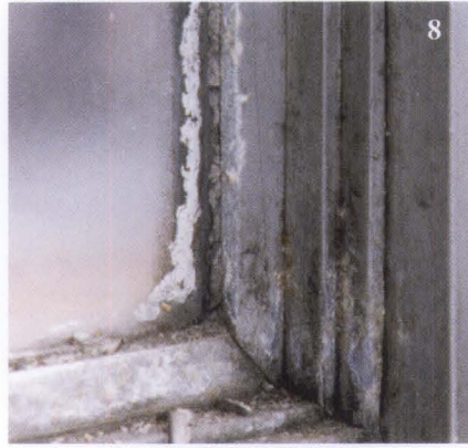
Figures 7 and 8. Aluminum corrosion can appear as a white discoloration and forms on the surface as the protective oxide film breaks down, as seen in these 60 year old windows in the PSFS Building, Philadelphia, before they were replaced. The small dark bumps are where surface dirt, grime, and pollution particles collect. Over time, pits form beneath these dark areas as the surface continues to corrode. This corrosive action is further encouraged by foreign particles, such as dirt and chlorides, which hold moisture next to the surface. (Photo: Powers & Company Inc.) Figure 9. Some aluminum alloys are less corrosion resistant than others. Delamination, as seen on this aluminum railing in front of a window at the Folger Shakespeare Library, can occur when an aluminum-copper alloy is introduced and used in an outdoor setting. The original specifications called for aluminum and chromium, but were not followed.
