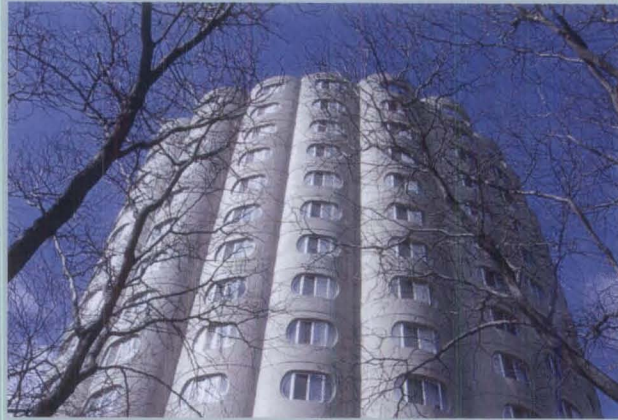
Figure a. One of two identical 16-story senior citizen apartment buildings within the Raymond M. Hilliard Center, each with 182 apartment units. The window openings are elliptical in shape and center on each reeded bay. (Photo: Holsten Real Estate Development Corp.)
