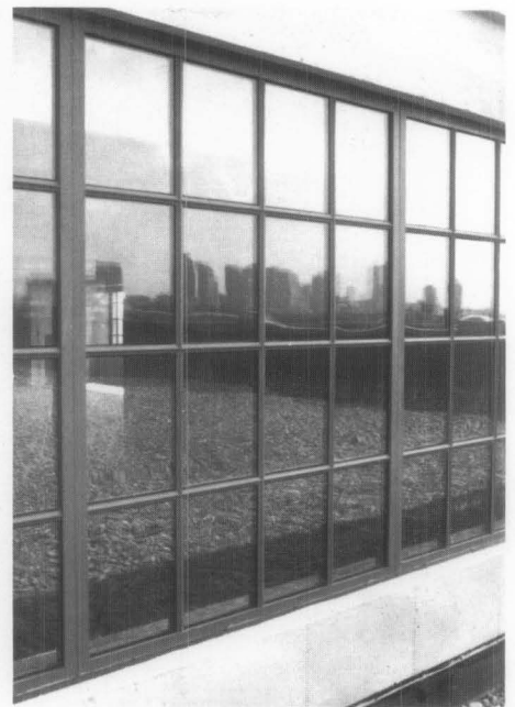
Figure 7. Despite the difficulty encountered with proper glass sizing and spacer alignment in the sealed insulating glass, the end result is an innovative window that is both aesthetically pleasing and closely matches the historic appearance of the original steel design. The slight encroachment of the bronze spacer onto the visible glass area is not readily detectable from general view. Photo: Charles Fisher
