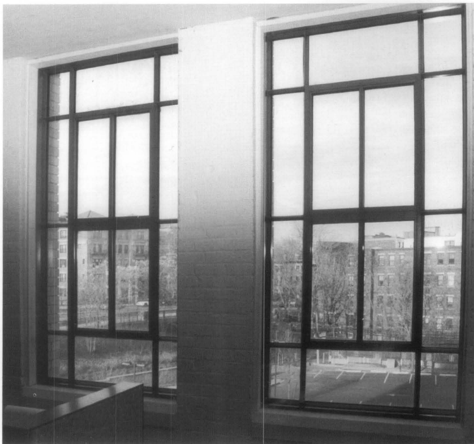
Figure 9. The interior profiles of the original windows were accurately reproduced in the aluminum replacement units. Photo: Bruner/Cott & Assoc., Inc.
