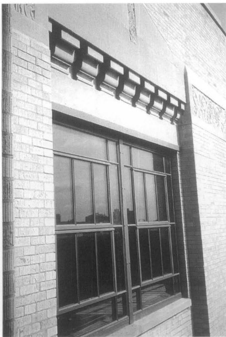
Figure 7. Installed replacement window. Photo: Bruner/Cott & Assoc., Inc.
