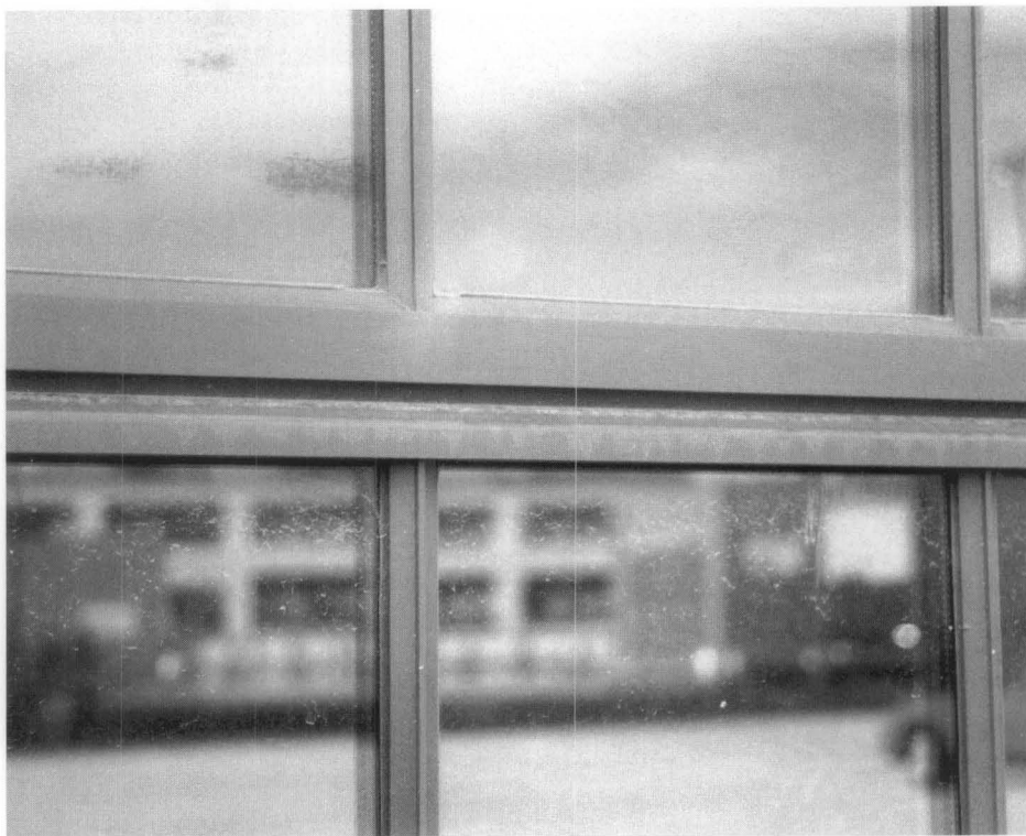
Figure 8. A close up view of the replacement window showing the replicated ventilator drip cap and narrow muntins. Photo: Bruner/Cott & Assoc., Inc.
