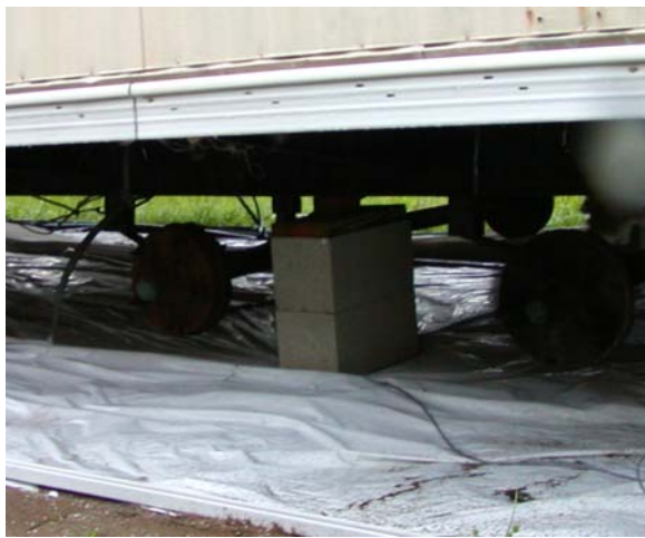
Figure 2 Ground Cover installed
