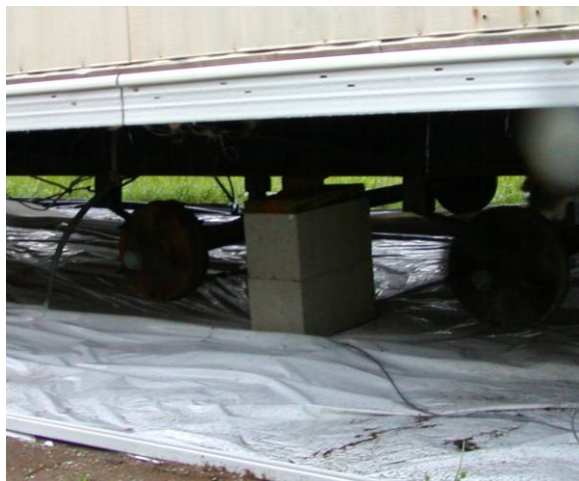
Figure 2 Ground Cover installed
