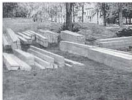
Showing Simple Plan of Laying Out Materials
