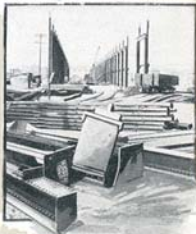
Readi-Cut System of Construction
